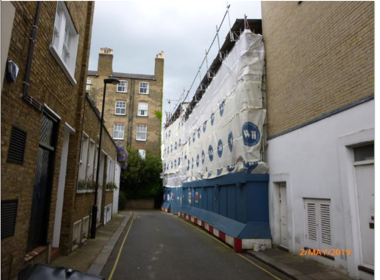
View from Bridstow Place towards Hereford Mansions
